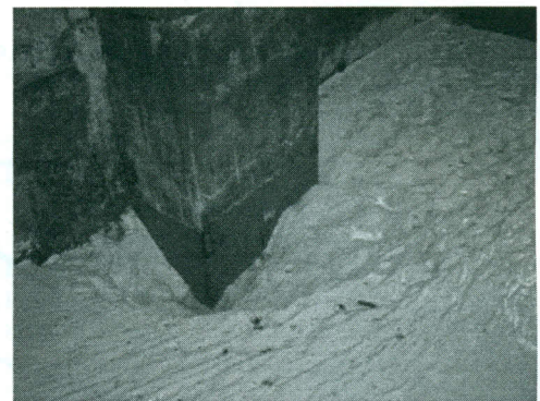
Figure 7 Eroded clay bed, no downstream deposition
